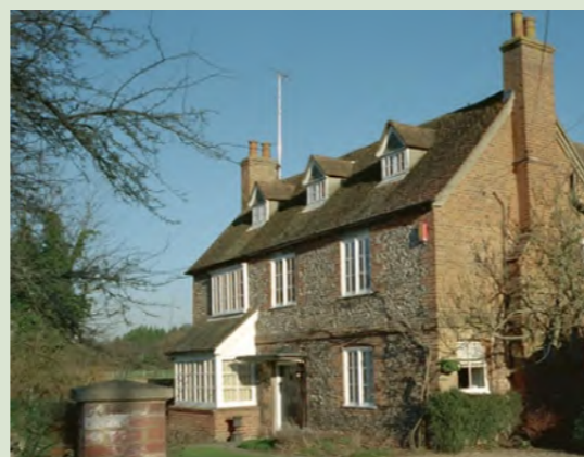
Figure TG9 - Well House - Grade II listed
