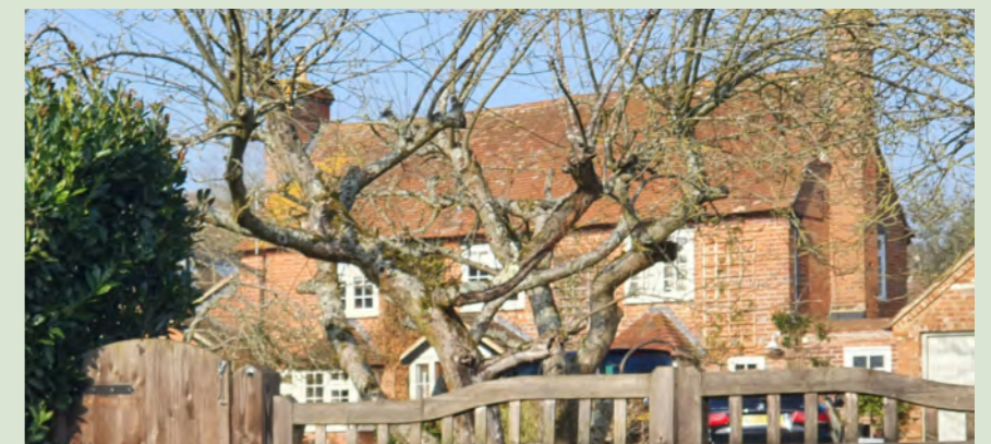
Figure GC9: The former Old Crown Public House - now a dwelling
