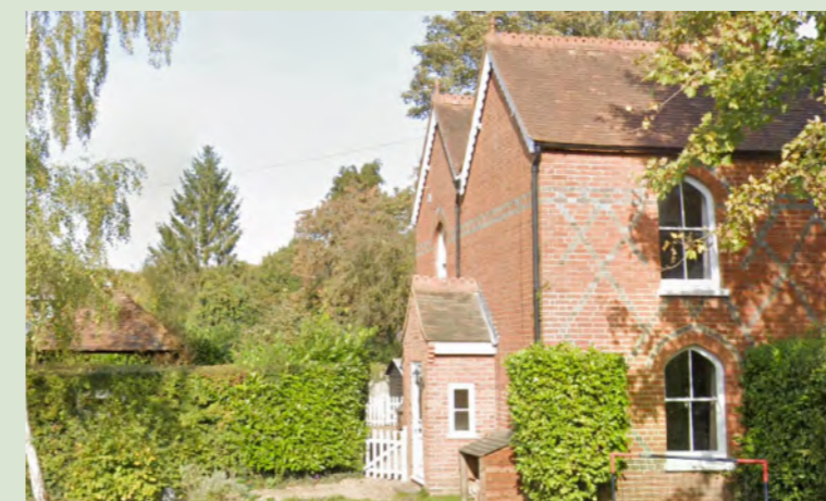
Figure GC5: Well Cottages - local red brick and plain clay tile with decorative brick work. The roof of the village well can be seen to the left of the dwelling
