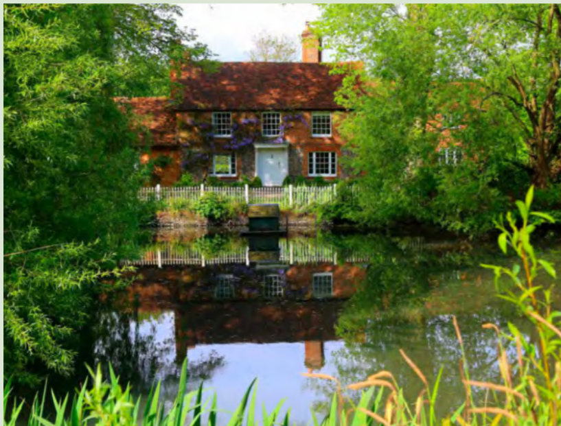
Figure KE1: View over the village pond to Pond House (Grade II listed)
