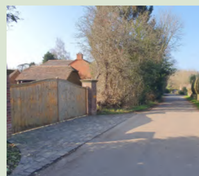
Figure GC28: block paving and tall gates can have an urbanising effect
