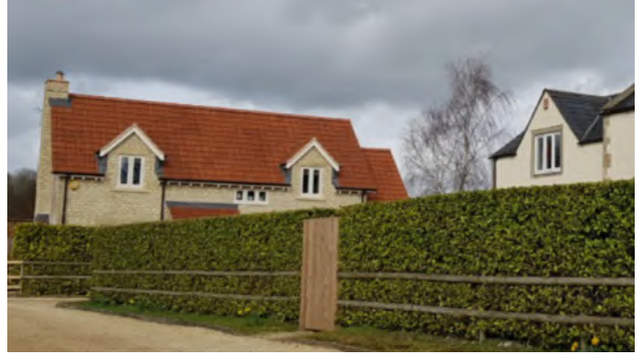
Careful consideration should be given to high quality materials and the level of detailing to add interest
