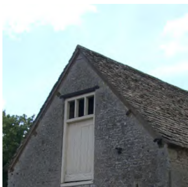
Retaining the existing hay doors contribute to the barn character
