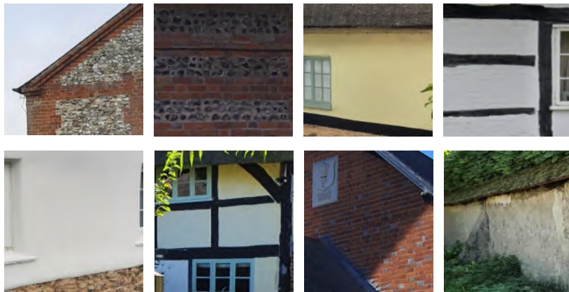
OW.I - WALLING MATERIALS - Timber frame with brick / Cob infill. Decorative brickwork detailing, string courses, quoins / dressings Flint panels and courses between brickwork
