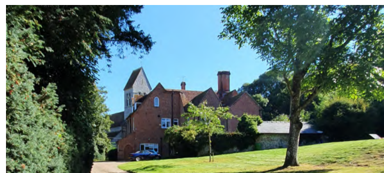
The Old Rectory - 18 th Century - local brick with blue headers and plain clay tile roof. Decorative brickwork and gable detailing as well as feature chimney stacks. Building set deep into the plot accessed by long gravel drive.
