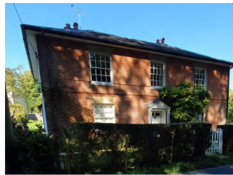
Foresters (GII) is an early 19 th Century house - local brick with string course detail and slate roof.
