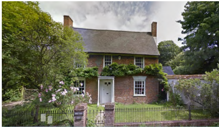
King's Farm was built in 1738 with later additions in 1832. It is Grade II listed farmhouse constructed of local brick with ornamental blue headers and a slate roof. To the rear of the property are two further Grade II listed buildings - a barn and a granary both constructed in weatherboarding. A cob and flint boundary wall separates this farm from the neighbouring Northern Farm to the east.
