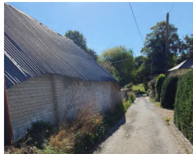
Grange Cottage (GII) 18 th Century Cottage- local brick with blue headers and flintwork to side elevation. Part thatch and part plain clay tile. Attached thatched and weatherboarded barn (GII)
