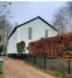
The Wallop Baptist Chapel (Chapel House) (GII) dates from 1841. It is of significance due to its construction of rendered cob with a slate roof and decorative detailing including stucco quoins, in addition to the cast iron gothic windows.
