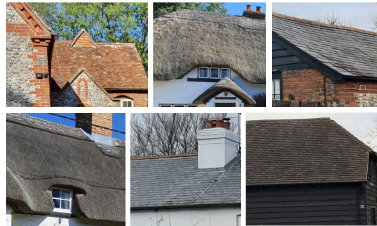
OW.II - ROOF MATERIALS AND FORM - Simple roof forms - gables, hipped and half hipped
