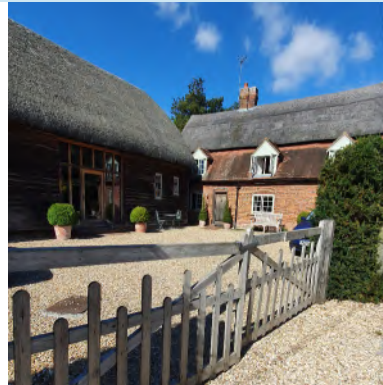
Grange Cottage (GII) 18 th Century Cottage- local brick with blue headers and flintwork to side elevation. Part thatch and part plain clay tile. Attached thatched and weatherboarded barn (GII)
