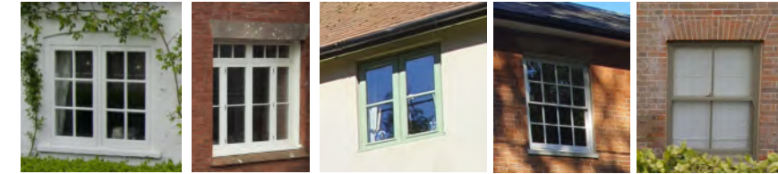
OW.III - WINDOWS & DOORS - Timber cottage casement windows - triple pane/ double pane - arch topped and sliding sash windows. Lighter paint colours are preferable
