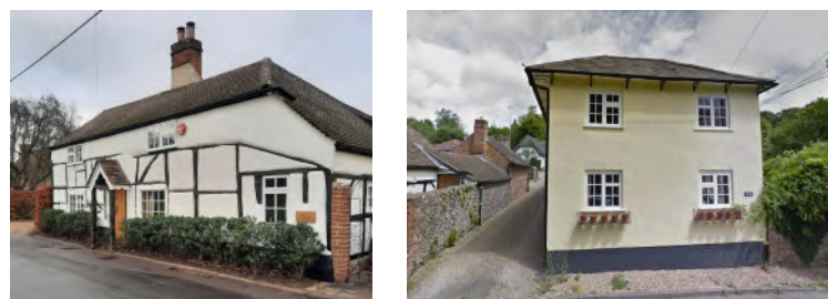
(Left) Wayside Cottage (GII) 17 th Century Cottage - Timber-frame with plaster infill and plain clay tile roof - hipped with swept outshot.
