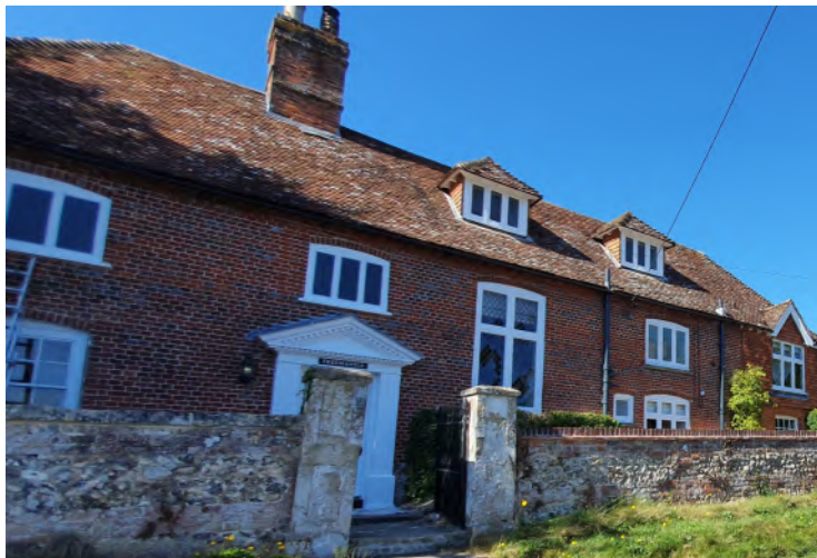
Freemantle (GII) is a mid 18 th Century house - red and blue header bond brick with plain clay tile roof. It has a number of outbuildings including a GII listed barn. It was named after its owner Mr John Freemantle
