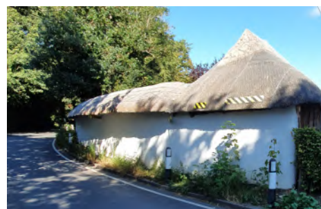
The wall surrounding The property known as The Walled Garden is one of a number of listed cob and thatched walls in the village
