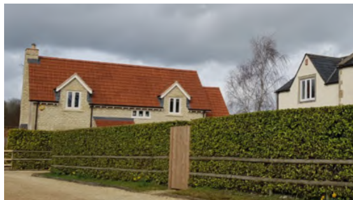
High quality materials. Dormers are low key and break the eaves line
