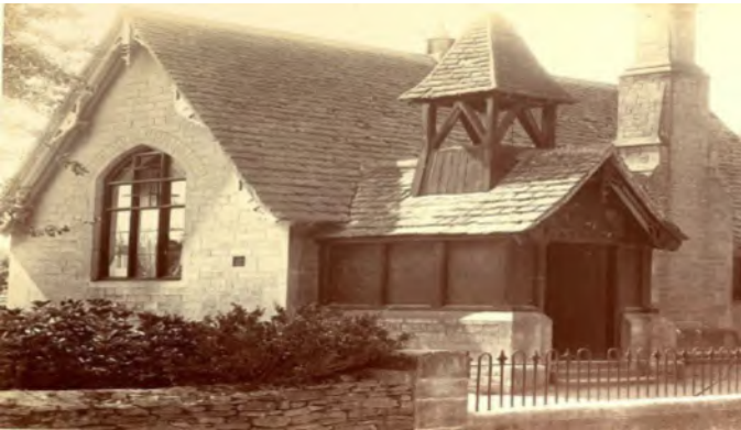
The National School built in 1850 as taken in 1905 - now a private dwelling
