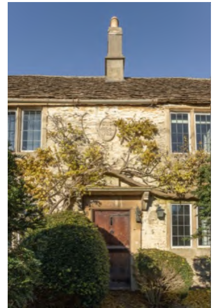
Ross Cottage dates from 1782 - rubble stone with stone slate roof
