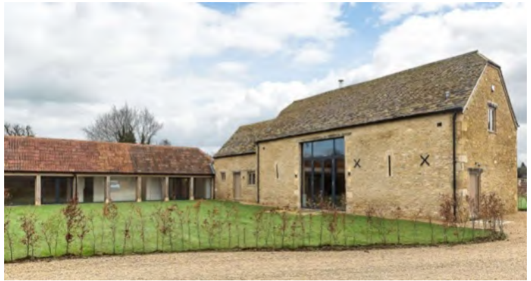
Barn at Arms Farm - recently converted to residential use. Late C18, rubble stone with stone slate half-hipped roof - south side hipped projecting cart-entry
