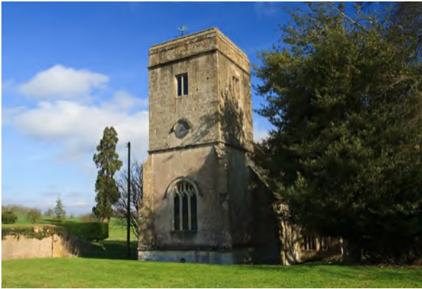
Church of St James - Draycot Cerne Grade II* - c1300 with C16 west tower, altered in mid C19, rubble stone, ashlar tower, stone slate roof
