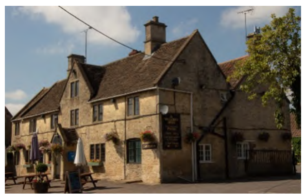
Wellesley Arms Public House - mid C18, rubble stone with stone slate roof,
