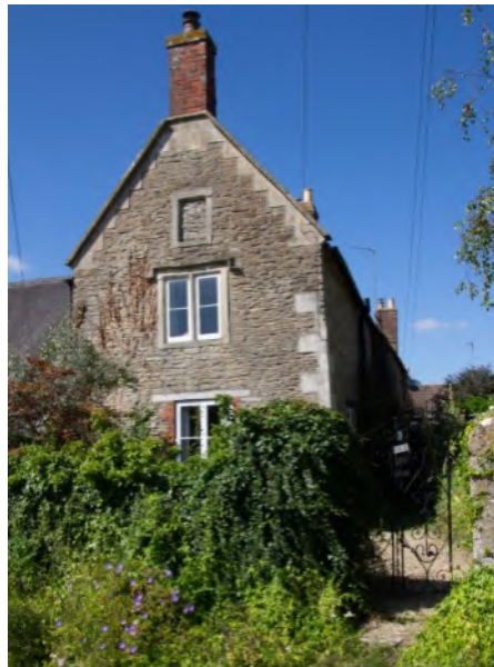
68/ 70 High Street - Pair of houses, C18, roughcast rubble stone with pantiled roof
